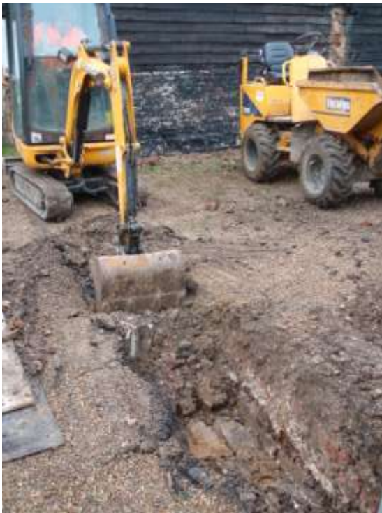
Plate 3. Cutting of first trench (Day 1)
