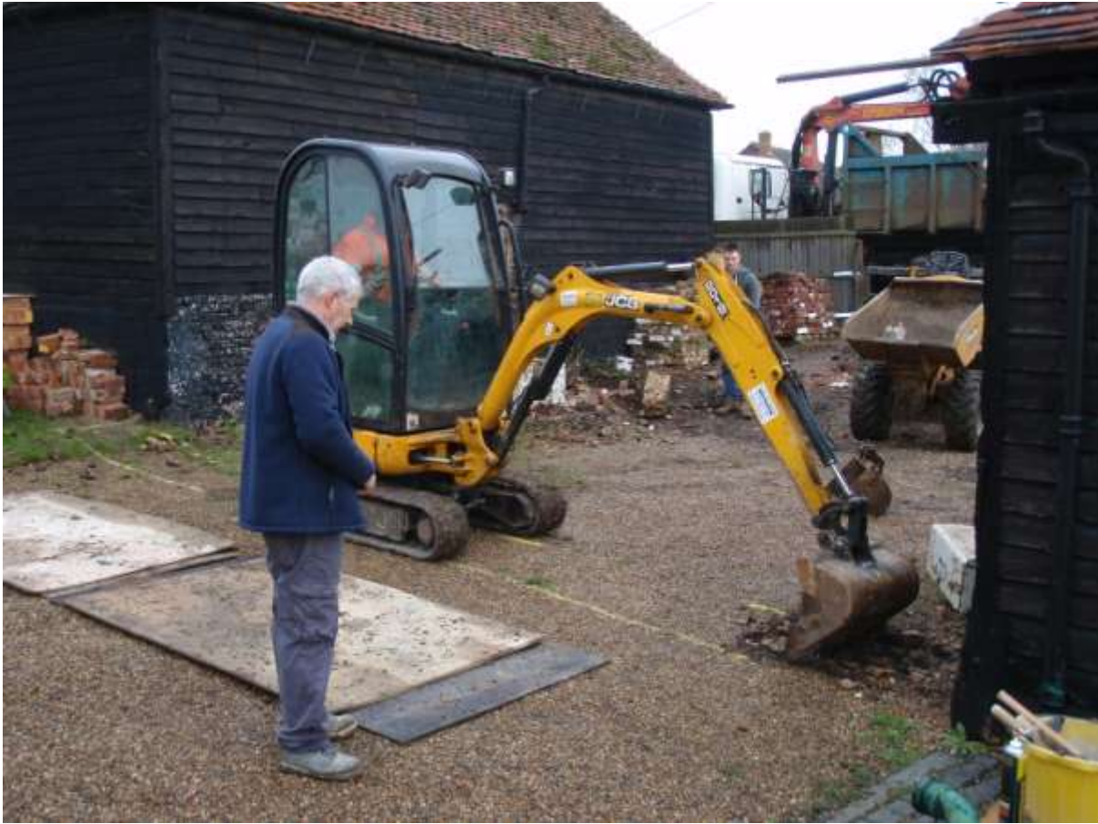
Plate 2. General view of site (looking NW)
