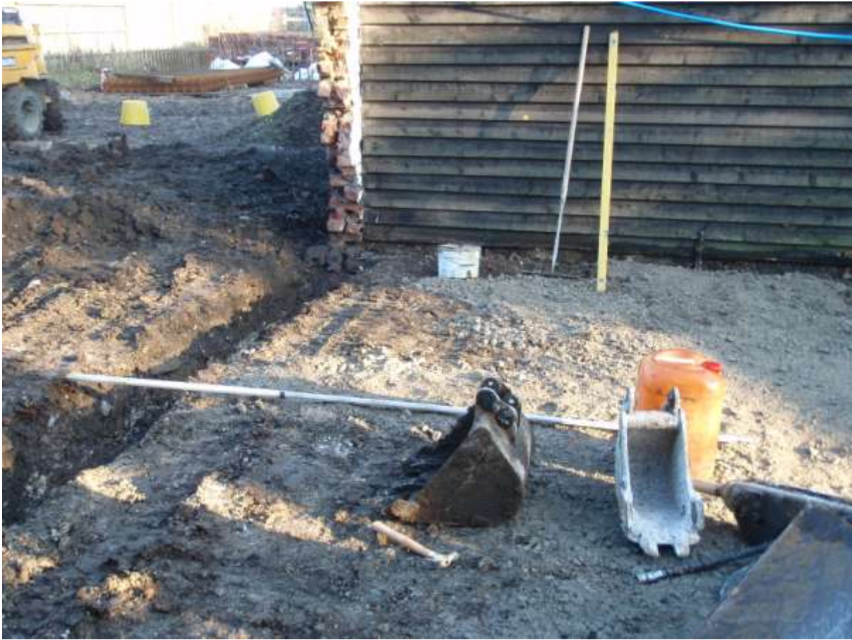
Plate 6. View of trenching (Day 2)
