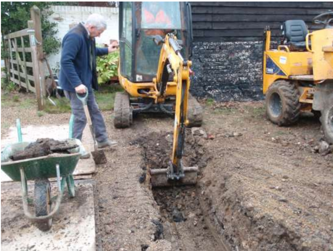
Plate 5. Close up of trenching (Day 1)
