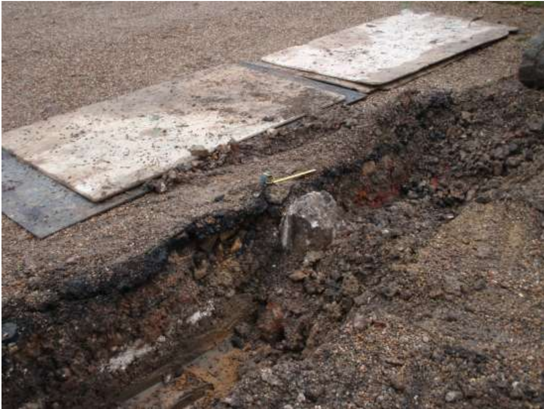
Plate 4. View of trenching and stone stylobate of previous open fronted barn (Day 1)
