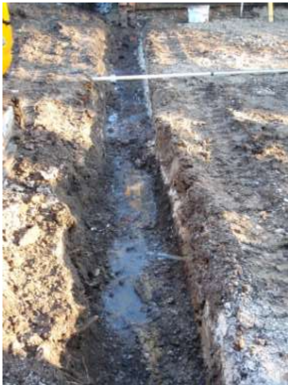
Plate 7. Completed trenching (Day 2)
