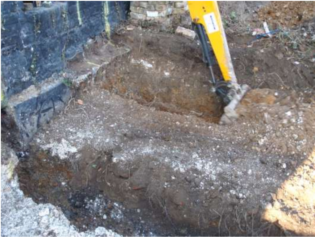
Plate 8. Section of drainage trench (Day 2)
